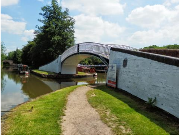
The 1830s iron bridge carrying the towpath over the original line of the Oxford. This was bypassed when the Oxford was shortened, and became a busy Arm of the Grand Junction with a boat builder and other facilities there.
