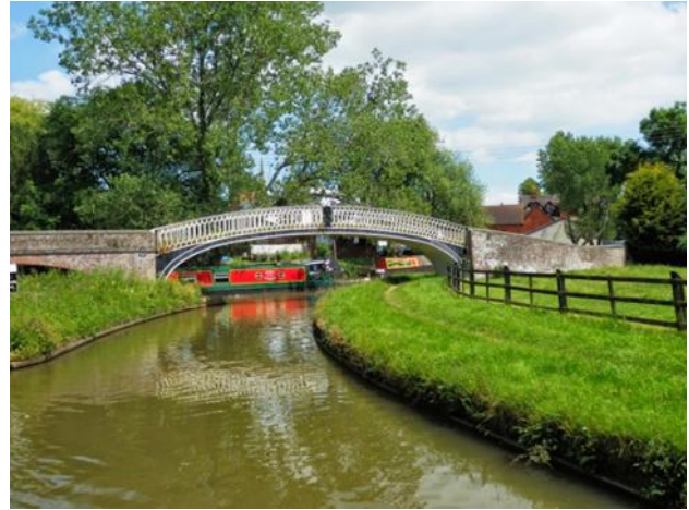
Another 1830s Horseley Iron Bridge used to deal with the changes to the Oxford's line when it was straightened. This carries the Oxford's own towpath over the new junction.
